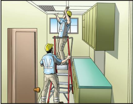
Step platform deployed for checking the ventilation system in a room where there is restricted space to accommodate a typical working platform.
